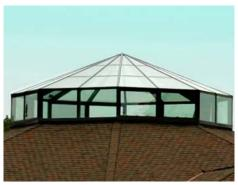
Thermally broken frames to stop exterior metal from touching interior metal, significantly reducing the transfer of heat and cold.
